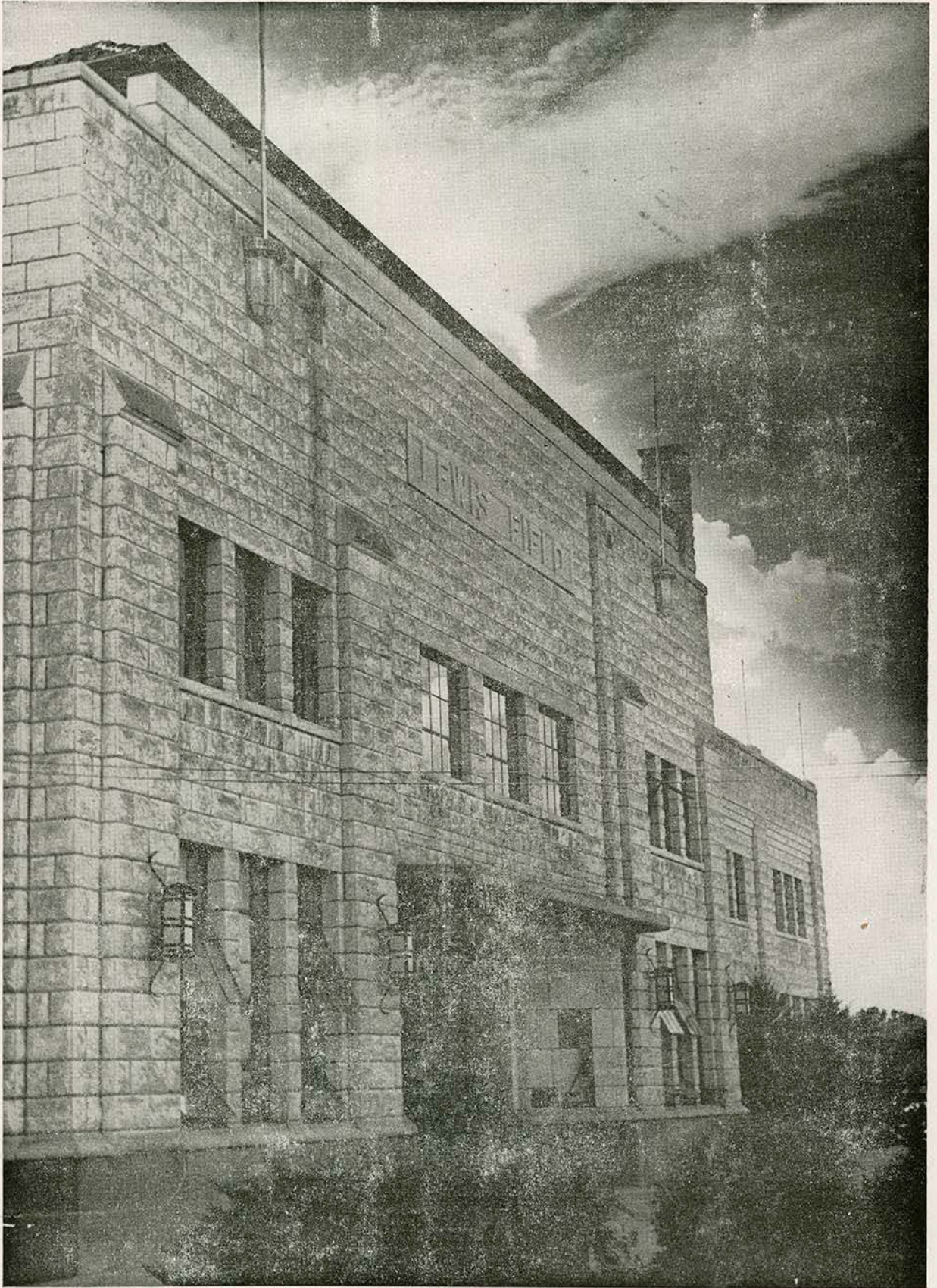
LEWIS FIELD STADIUM
